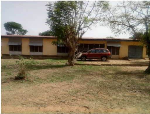
Plate 4: Case Study1 South Elevation Source: Fieldwork (2023)
