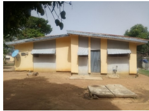
Plate 5: Case Study1 East Elevation Source: Fieldwork (2023)
